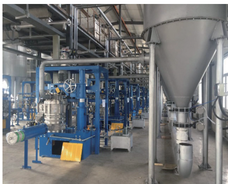
図4 F-430S 納入例 Fig. 4 Faculty machine F-430S photo
