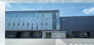
New Osaka factory
